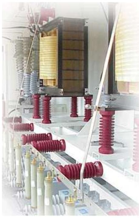
Above two pictures shows how NEPSI interconnects components with Silver or Tin-plated Copper Bus Bar. This method of interconnection is not prone to failures associated with forces during capacitor bank energization. Over the life of the equipment, air provides the best insulation medium as it does not allow for tracking or treeing that is common with solid dielectric cables. See the following link for further information on Phase and Ground Bus System.
