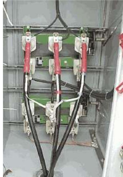
The above pictures show a couple of our competitor's incoming compartments and extensive use of "tiger cable" or jumper cable". Note the long runs of cables, and places where cable fatigue can occur. Also note lack of steel barrier between incoming compartment and capacitor compartment and the use of tie wraps to hold current transformer secondary wires. Remember that tie wraps can be expected to fail within one to two years.
