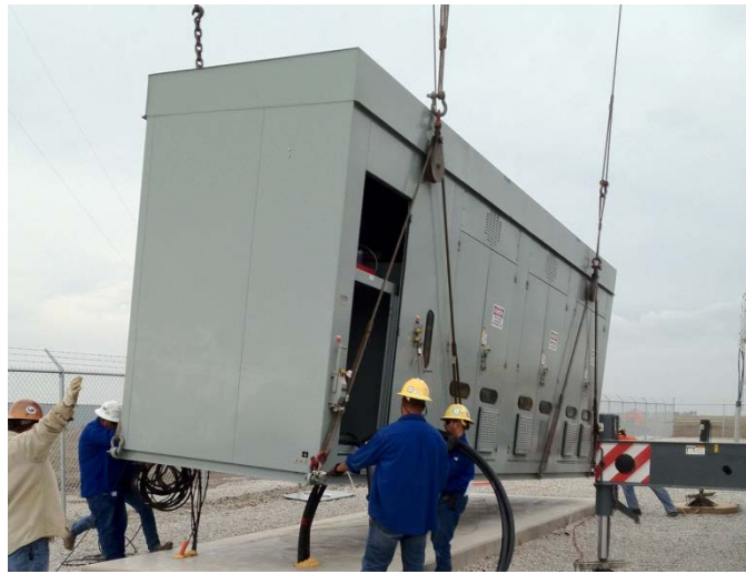
Figure 3 - actiVAR™'s are Shipped Fully Assembled and Ready for Interconnection. Enclosures are designed for indoor and outdoor application.
