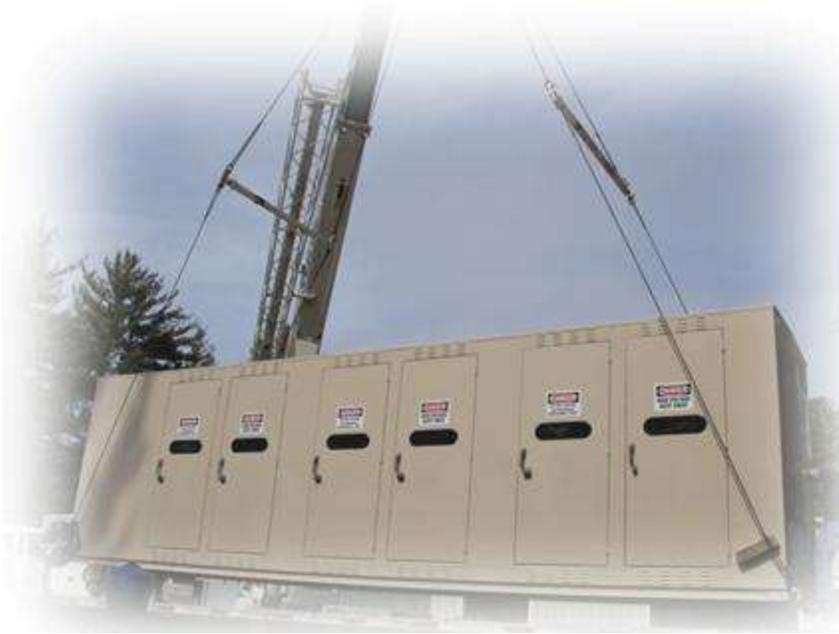
Figure 8 - Picture to left shows the 18 MVAR 3 Step 3 stage automatic capacitor bank being loaded for shipment to the City of Burbank. The bank was of all stainless steel construction and painted per the customer's requested color.
