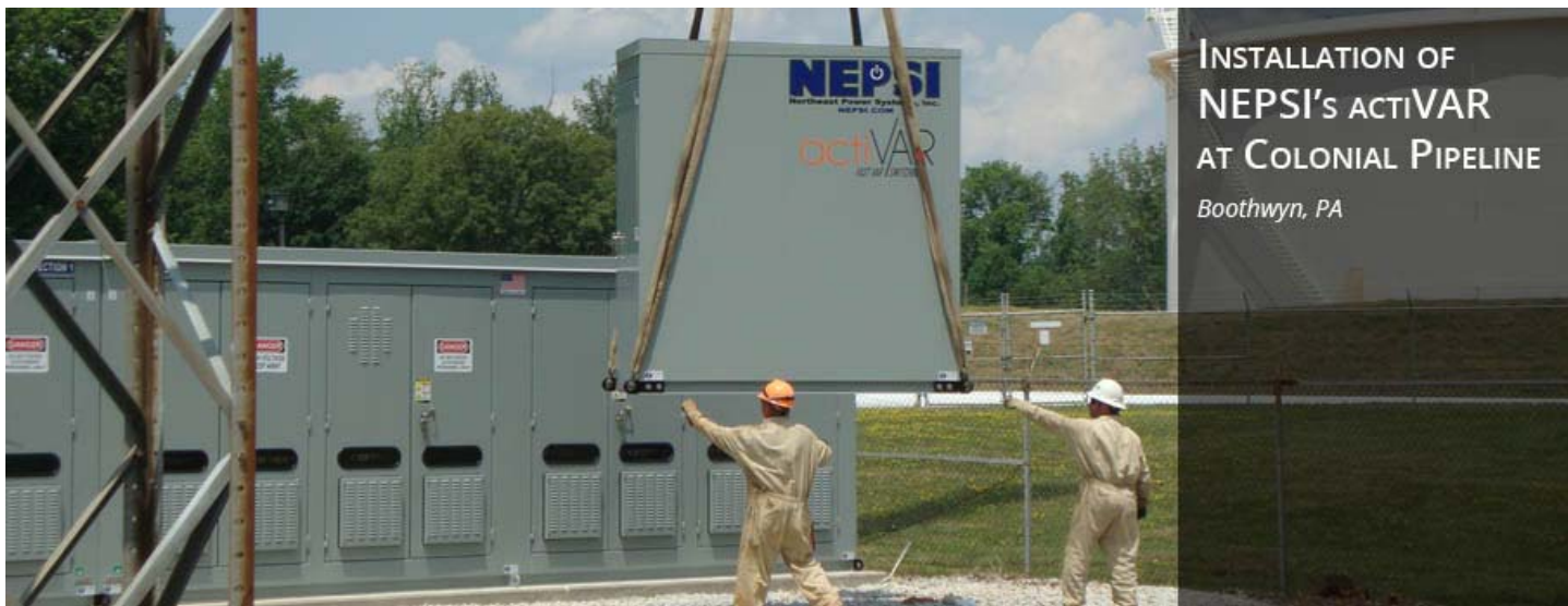
Figure 3— (below) actiVAR™ being installed in CPC’s substation. The actiVAR™ comes fully assembled, tested, and ready for inter-connection.
