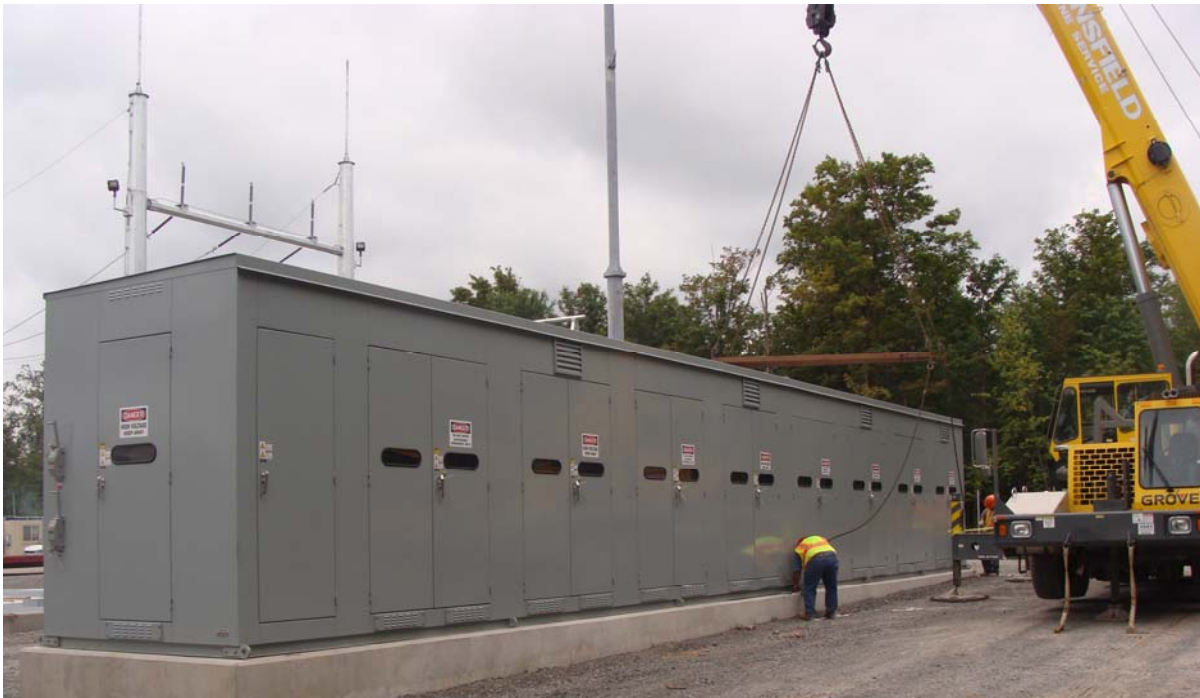
Figure 9: Typical Harmonic Filter Bank Specified by Northeast Power Systems, Inc.
