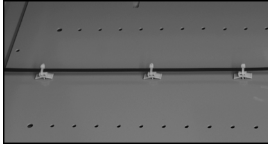
Figure 2.26 Jacketed-Fiber Installation Example
