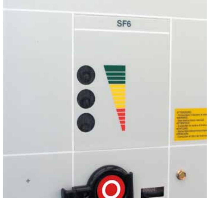
SF6 control device with 3 LEDs.
